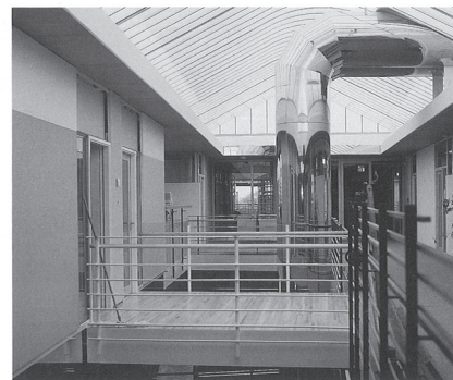
View of a corridor showing top-lighting.
